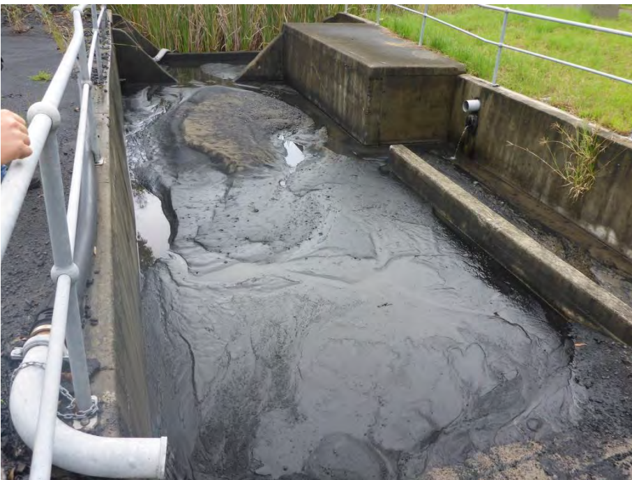
Photo 2 Material to be removed from sumps
