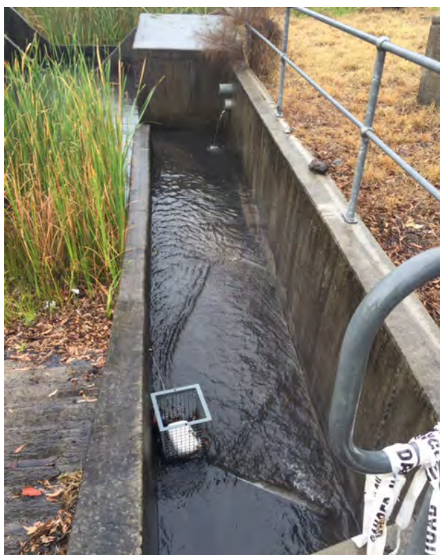
Photo 1. Flocculent block located adjacent the coal stockpile area.
